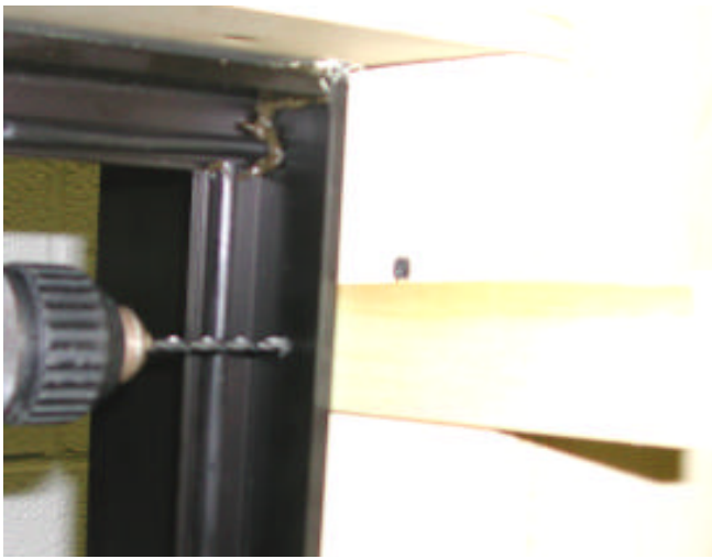
PREDRILL AND APPLY ANCHORS
