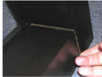
CAULK AND SMOOTH EXTERIOR SURFACE OF PANNING
