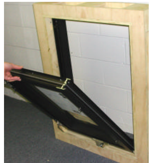
TILT WINDOW IN FROM INTERIOR
