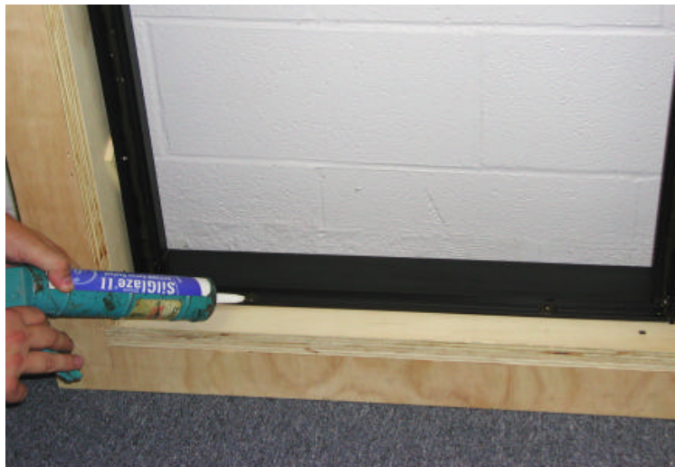
APPLY CAULK OVER ALL FASTENERS
