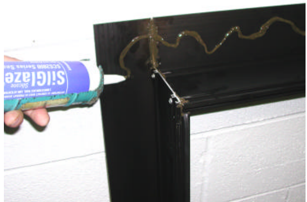
APPLY CAULK TO INSIDE LEG OF PANNING
