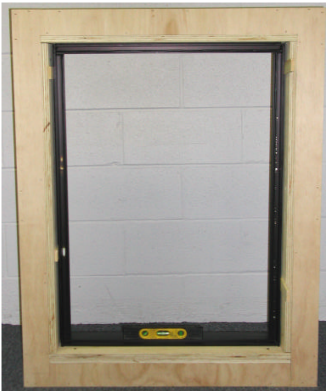
SLIDE PANNING INTO OPENING SHIM AND LEVEL
